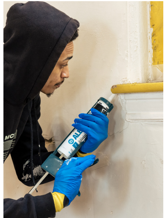
The weatherization process
